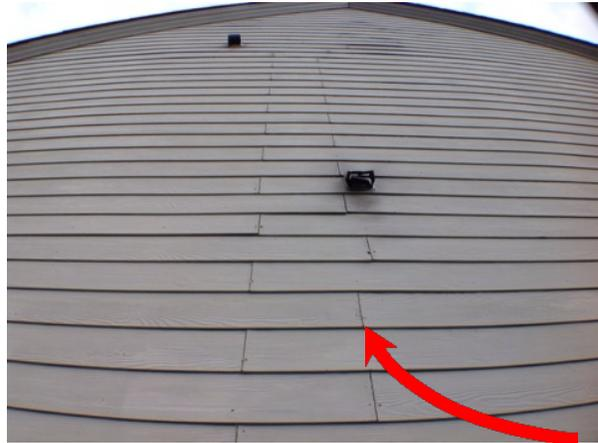
Walls/Siding/Trim - Caulked joints of siding are cracking.
