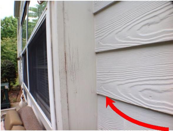
**Walls/Siding/Trim** - Caulk is separating in rear window bump out.
