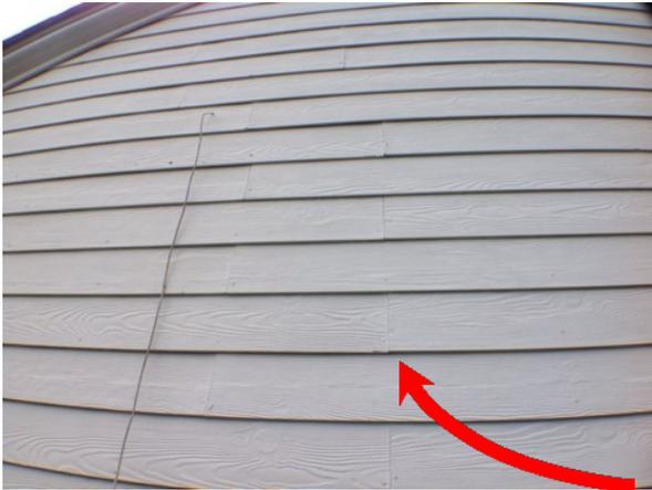
Walls/Siding/Trim - Caulked joints of siding are beginning to crack.
