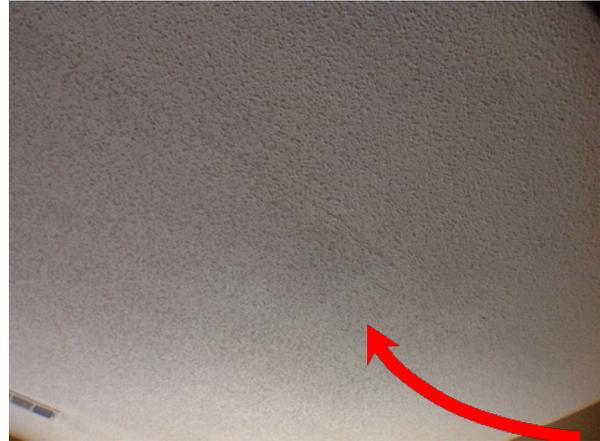
**Ceiling** - Slight cracking in what looks like an old patch.
