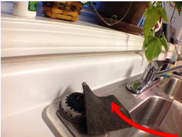
Counter Top/Back Splash - Caulk discolored and cracking behind the sink.
