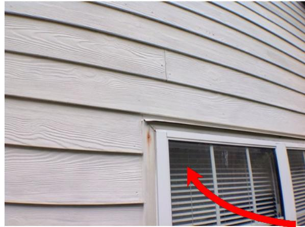
**Walls/Siding/Trim** - Rear window trim is cracking and discolored.
