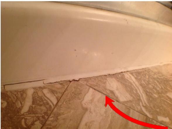
Shower/Fixture - Cracking Caulk on exterior of shower tray.
